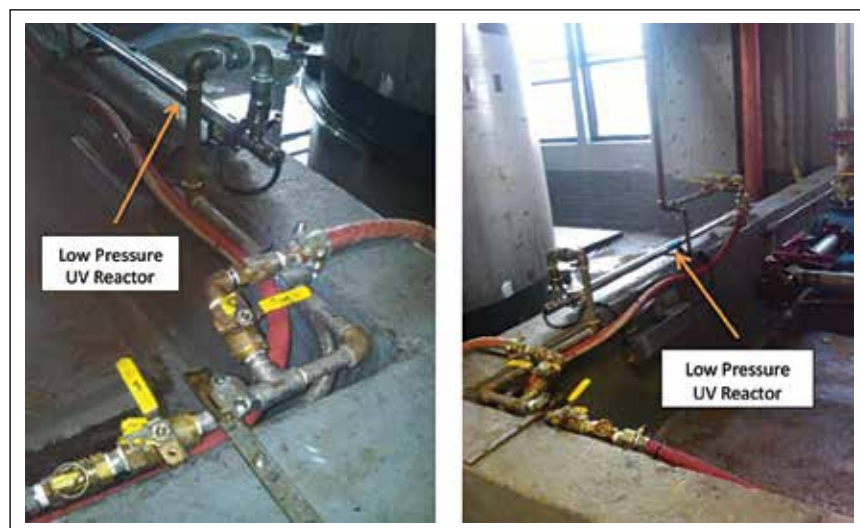
Figure 2. Photographs illustrating the installation of the low pressure lamp UV pilot reactor in the Medium Invert Syrup production system
